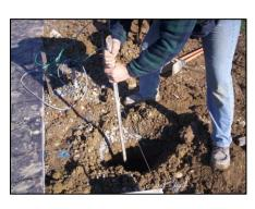
Fence installation is no different from any other construction project. Fence posts require a solid base so there is no settling. Weather the hole is dug by hand or with a machine; always remove the loose soil from the bottom and tamp it firm.
