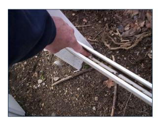
Take the replacement rail and slide it into the hole of one of the posts on the section that is being repaired, push it in till the notches are inside the post and the rail will not pull free. Then set the other rail end on the top of the adjacent post as shown below.
