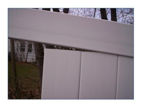
At this point, the top rail is carefully slid off the top of the post where it was placed earlier and allowed to rest on the pickets that have just been installed.
