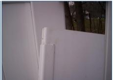
Holding the picket on a slight angle, slide the bottom of the picket into the slot of the lower rail while being mindful that its bottom edge on the opposite side may get caught on the lip of the rail. Very often the picket can be manipulated into place by wiggling it and applying downward pressure. If this does not work, a free hand can be placed between the pickets and used to force the bottom toward the installer while pushing down with the other hand.
