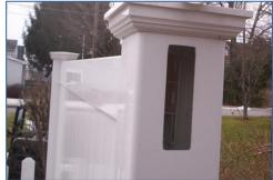
Once the rail has been cut and removed the pickets will drop if they didn't do so previously. The slot in the bottom rail should be cleaned of any debris so the pickets mate well. Using a rag or paper towel, dirt and grime can be pushed toward the rail opening in the post and be swept into it. The top rail can now be set up to reinstall the pickets.
