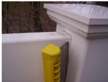
The tool is inserted into the gap between the rail and the post by holding it at the angle that allows the curved end to lay flush on the rail. When fully inserted, the metal will allow the tabs to slide past the inside edge of the post and the rail will come free.
