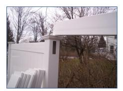
The slot in the bottom rail should be cleaned of any debris so the pickets mate well. Using a rag or paper towel, dirt and grime can be pushed toward the rail opening in the post and be swept into it. The top rail can now be set up to reinstall the pickets.
